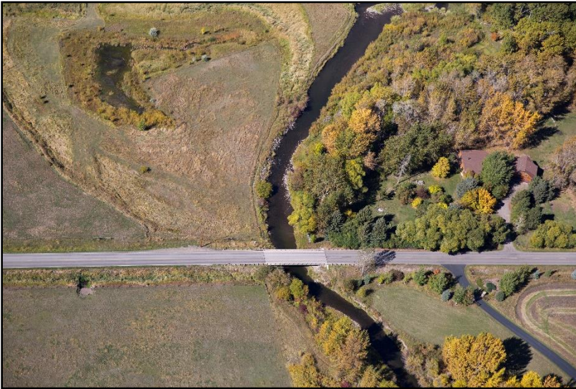
Figure 72. Manley Road bridge on September 26, 2016. (Kestrel)
