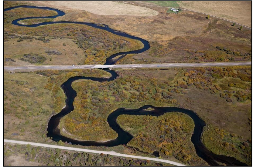
Figure 82. W Dry Creek Road bridge on September 26, 2016. (Kestrel)
