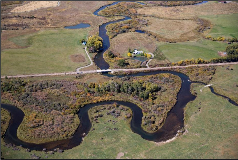
Figure 80. Swamp Road bridge on September 26, 2016. (Kestrel)
