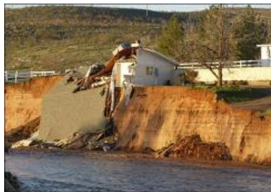
Figure 4. Yellowstone River home on high glacial terrace that was burned down in 1997 to prevent its undermining by the river.
