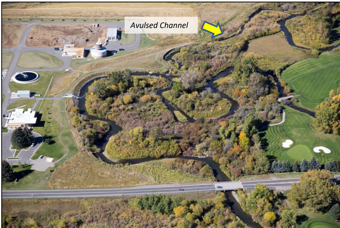
Figure 51. Reach EGR 6 showing avulsion site at Bozeman Water Treatment Plant (Kestrel).
