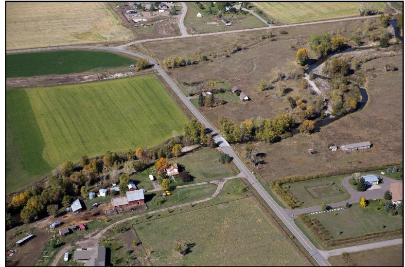
Figure 74. Airport Road bridge on September 26, 2016. (Kestrel)
