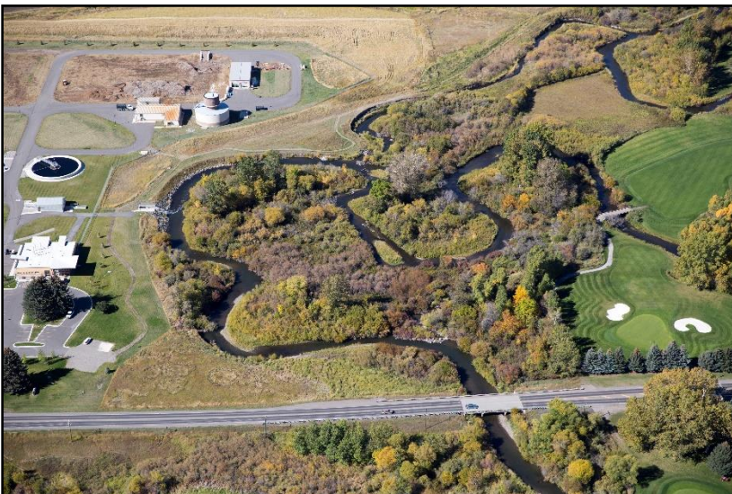
Figure 73. Springhill Road bridge on September 26, 2016. (Kestrel)
