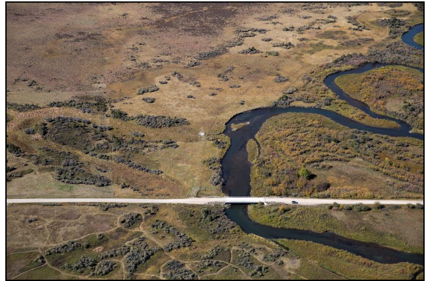
Figure 83. Spaulding Bridge Road bridge on September 26, 2016. (Kestrel)
