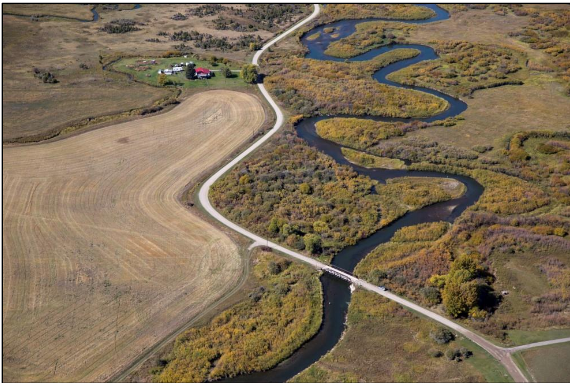
Figure 66. View downstream from Dry Creek School Road Bridge showing healthy riparian corridor (Kestrel).
