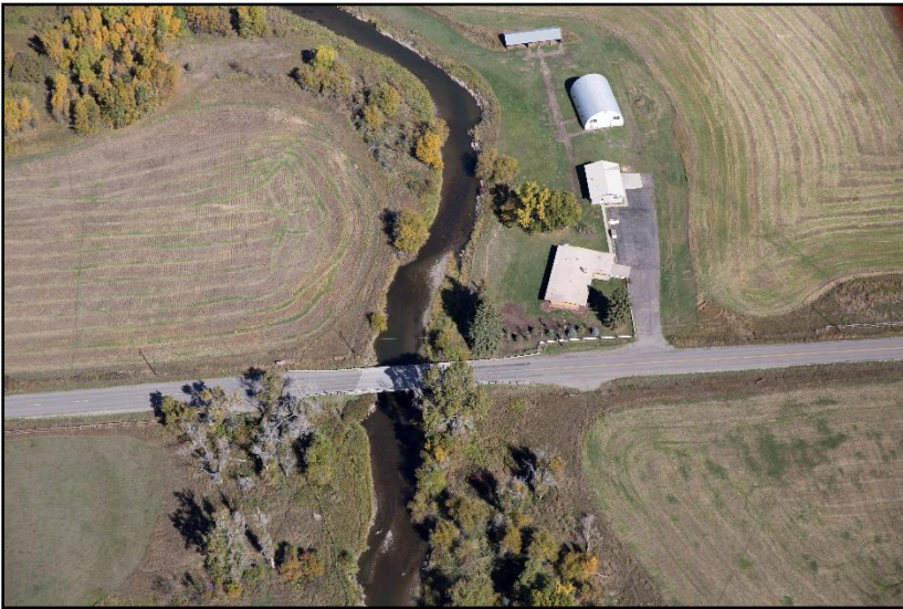
Figure 77. Penwell Bridge Road bridge on September 26, 2016. (Kestrel)
