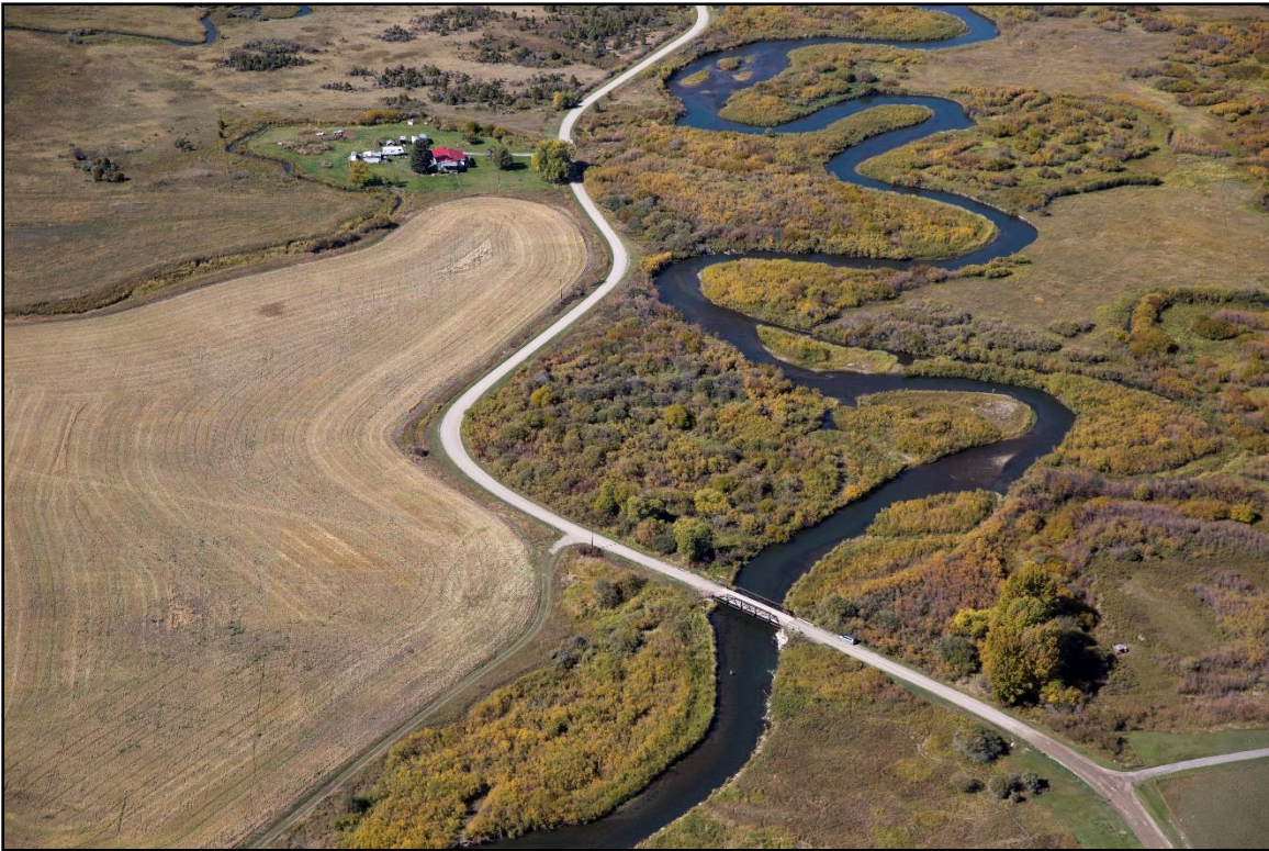
Figure 19. Right bank armor associated with the Dry Creek School Road bridge approach. (Kestrel)
