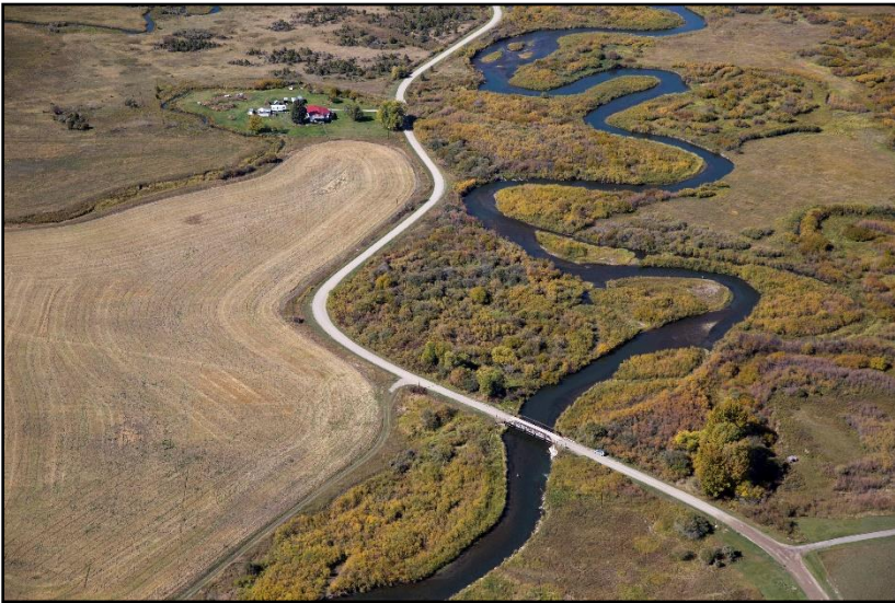
Figure 81. Dry Creek School Road bridge on September 26, 2016. (Kestrel)
