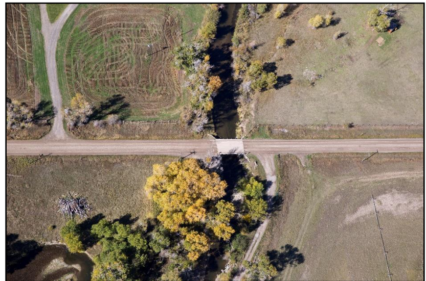
Figure 75. Spain Bridge Road bridge on September 26, 2016. (Kestrel)
